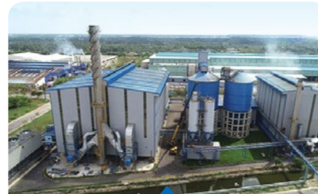
Co-Generation (Combined Heat Power)
