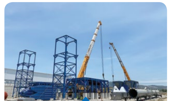
Steel Structure Erection
