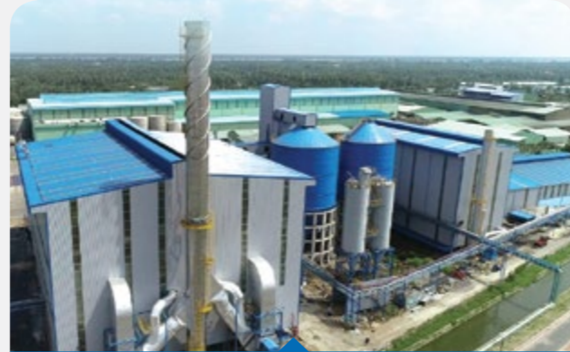
Co-Generation (Combined Heat Power)
